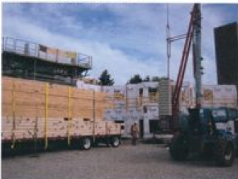
Truckload of wall panels
